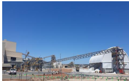
Greenbushes CGP2 Expansion project conveyor and stockpile shelter (2019)
