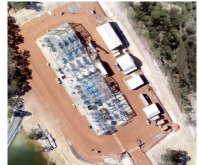
Waste Water Treatment Plant (2019)
